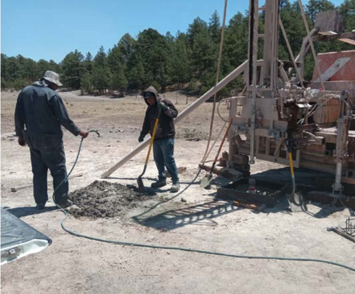
Drilling in Rosánachi
